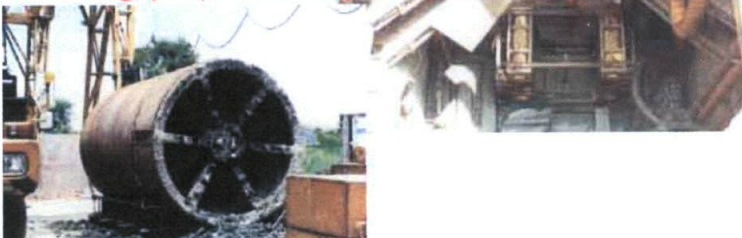
Slurry jacking head & Jacking pit(Rectangular)
